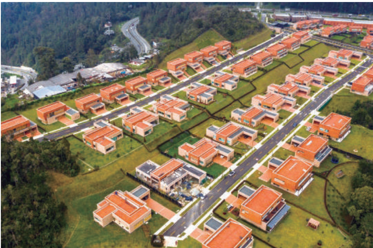
Lemont Country houses Envigado, Antioquia Covered with 10 mm Eterboard
