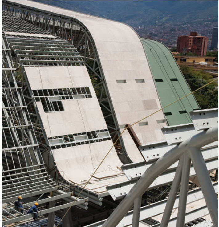
Construction: Coliseos Odesur, Medellín
